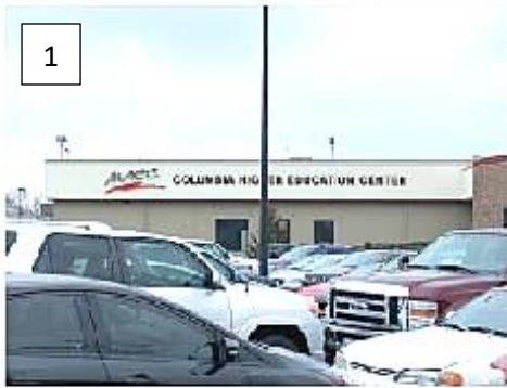
REMOVE AND DISCARD EXISTING SIGN
