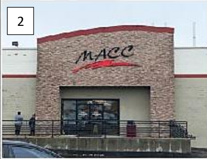
REMOVE AND DISCARD EXISTING SIGN
