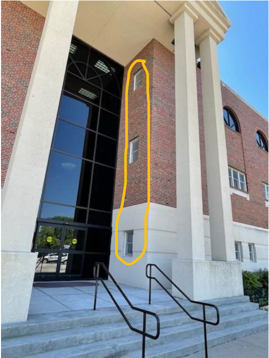
Front Corner of East Facing View
